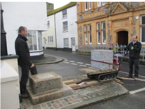
Finally, in October John and I started removing the setts and the 'garden'. By mid-November we had poured the foundation slab and laid the first two levels of granite. To significantly reduce overall costs these layers are reclaimed Westcountry granite, which John cut and faced.
